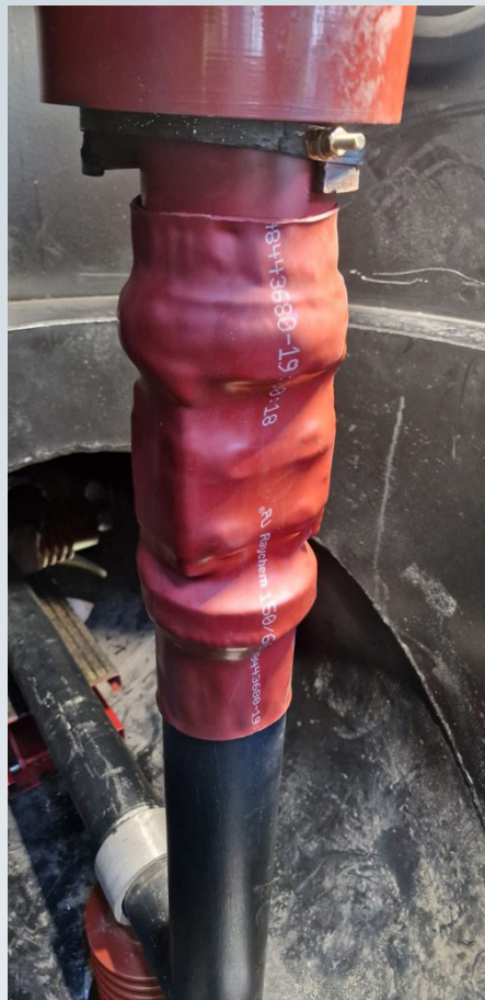
Figures 6 & 7 - Images showing revised conductor arrangement with central conductor now sleeved in heat-shrink busbar insulation material to act as primary insulation (Temporary Repair).
