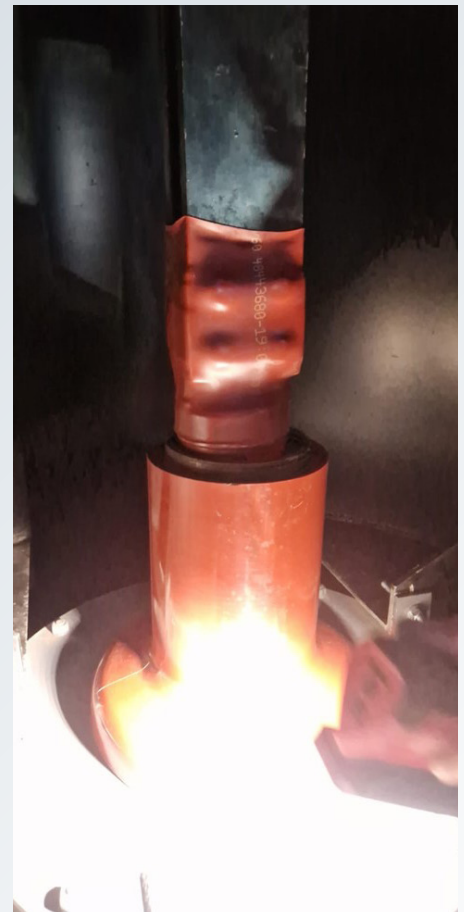
Figures 6 & 7 - Images showing revised conductor arrangement with central conductor now sleeved in heat-shrink busbar insulation material to act as primary insulation (Temporary Repair).
