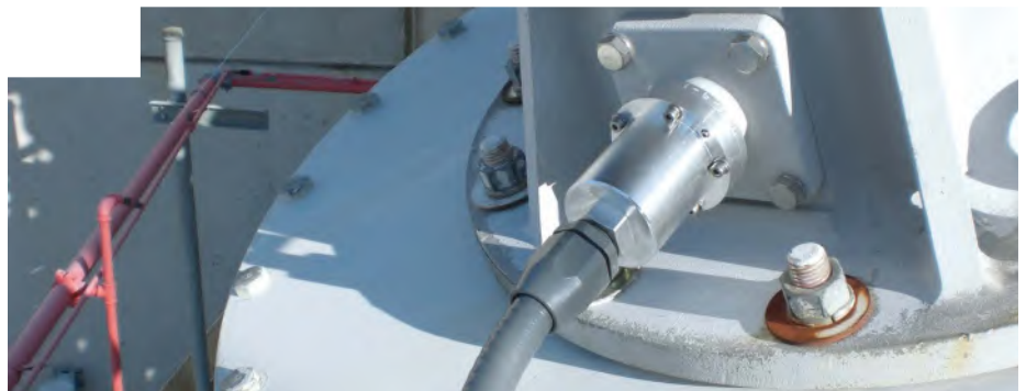
Figure 2. When installing a bushing monitor, it is important to ensure a secured installation and uncompromised contact with the test tap
