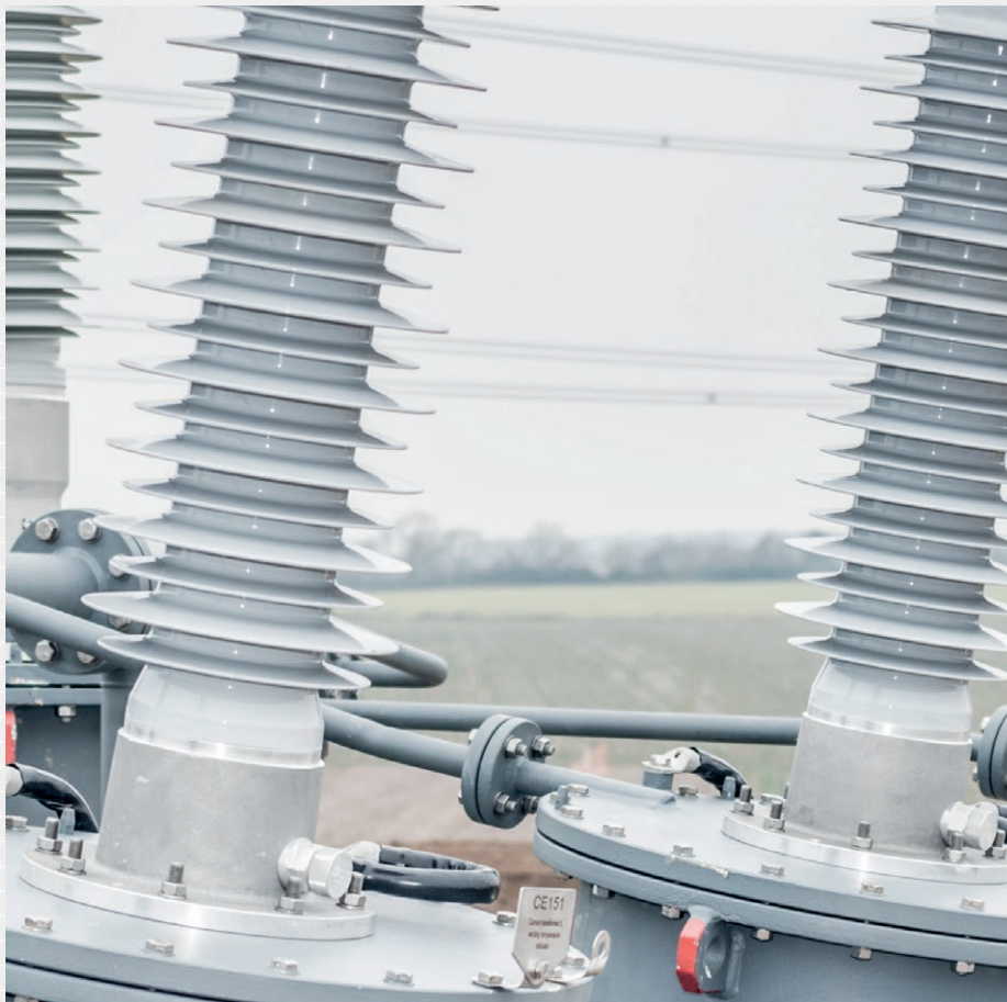
Figure 4 Pictures of two of the different designs of the BTP mounted on bushings.
