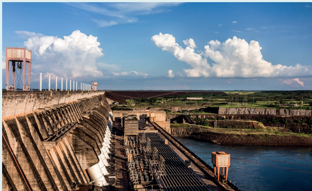
Figure 2. Overview of the Itaipu Power Plant
