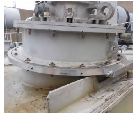
Figure 5. Top left: Clamp installed on transformer oil pump. Top right: Clamp installed around a top-mounted sudden pressure relay leaking oil at its mounting flange. Bottom left: Clamp being installed on the flange of a transformer access hatch. Bottom right: Transformer bushing turret clamp.
