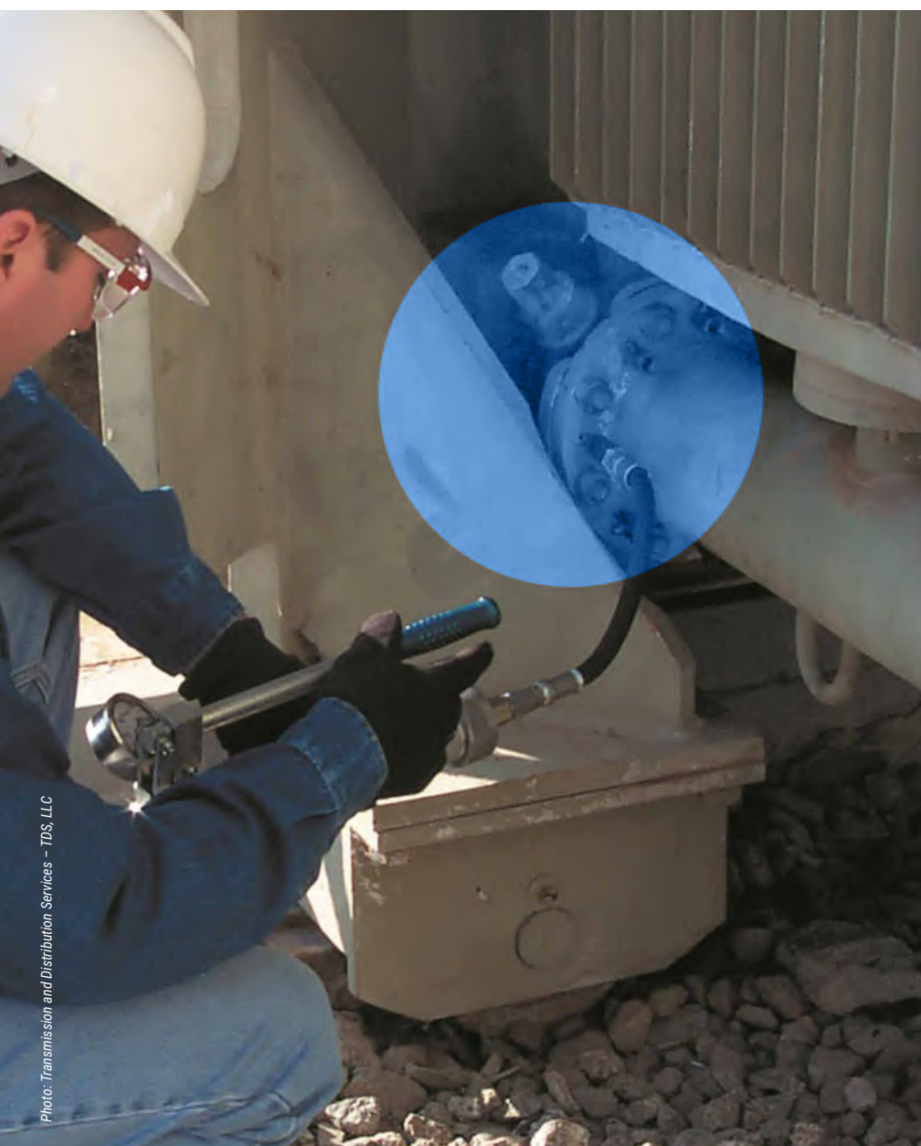
Figure 3. Drill and Inject technique: Online leak seal
