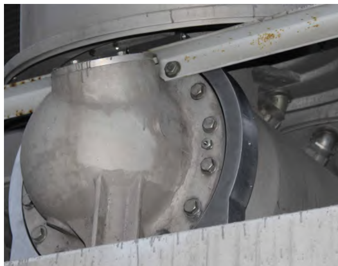
Figure 7. Left: Clamp on an EHV GCB bushing base. Right: Clamp enclosing on the end bell flange of an EHV GCB interrupter tank.
