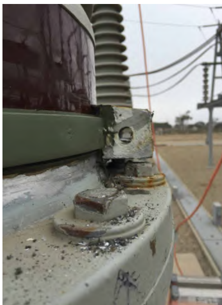
Figure 6. Left: Portion of clamp removed showing cured sealant. Top: Same repair, sealant cut away showing its flexibility.
