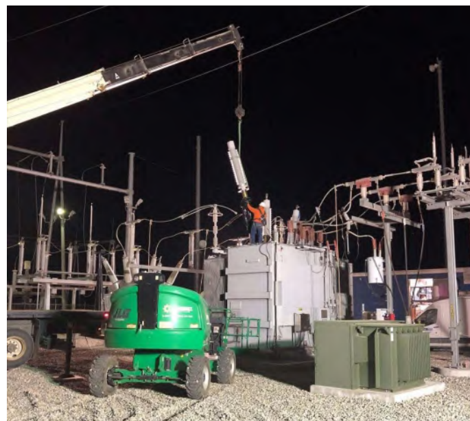
Figure 6. Night time H1 bushing replacement
