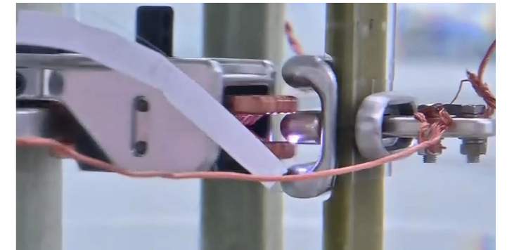
Figure 7: Discharge phenomenon when the tap changer performs a change-over switching in reverse phase between the contact bars
