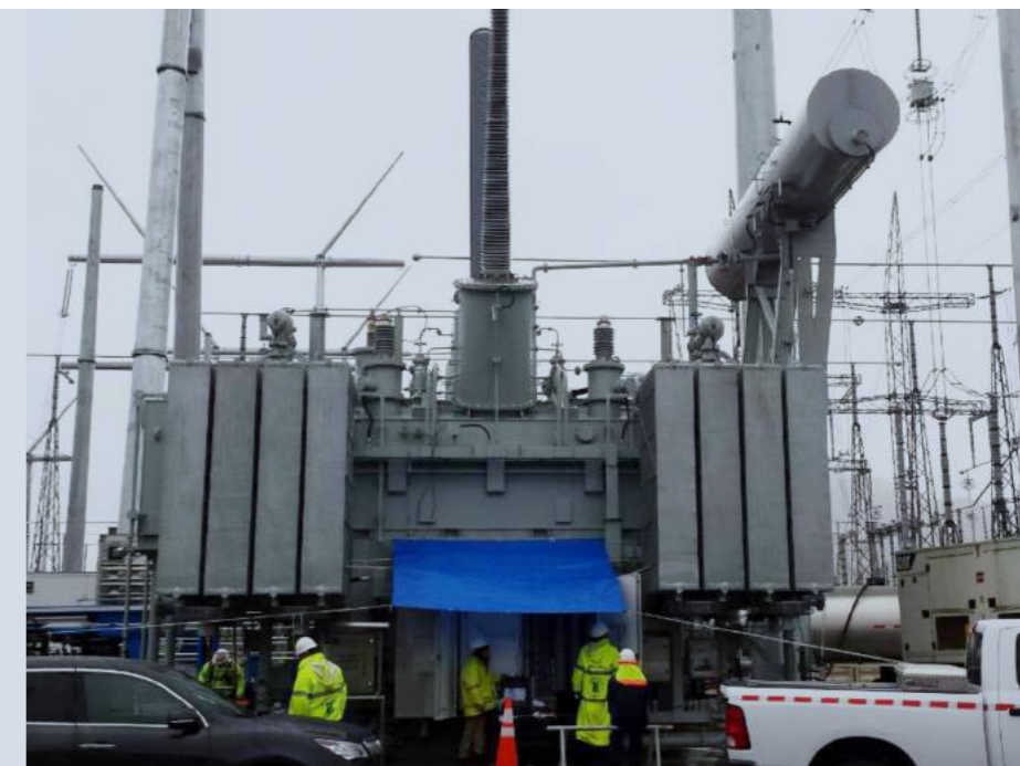
Figure 11: Picture showing the testing under energized lines and rainy condition
