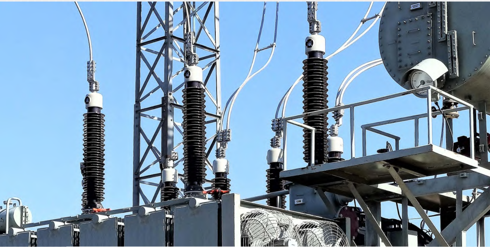
YASH MAKE 145 KV OIP BUSHINGS RETEOFITTED ON A TRANSFORMER TO REPLACE OLD SRBP BUSHINGS
