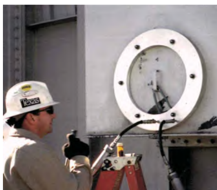
Figure 5. Top left: Clamp installed on transformer oil pump. Top right: Clamp installed around a top-mounted sudden pressure relay leaking oil at its mounting flange. Bottom left: Clamp being installed on the flange of a transformer access hatch. Bottom right: Transformer bushing turret clamp.
