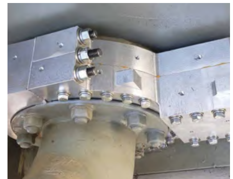
Figure 4. Top left: Open face flange and butterfly valve. This configuration will not support the Drill and Inject technique. Top: A three-part clamp butterfly valve. Bottom: A three-part clamp butterfly valve installed.
