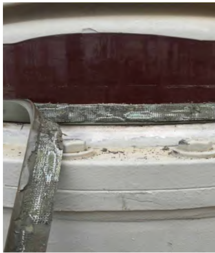
Figure 6. Left: Portion of clamp removed showing cured sealant. Top: Same repair, sealant cut away showing its flexibility.
