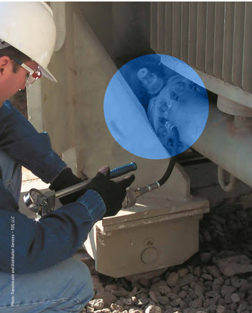
Figure 3. Drill and Inject technique: Online leak seal
