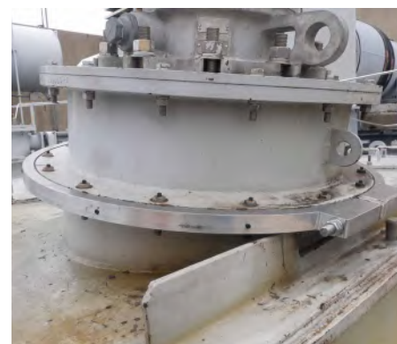
Figure 5. Top left: Clamp installed on transformer oil pump. Top right: Clamp installed around a top-mounted sudden pressure relay leaking oil at its mounting flange. Bottom left: Clamp being installed on the flange of a transformer access hatch. Bottom right: Transformer bushing turret clamp.
