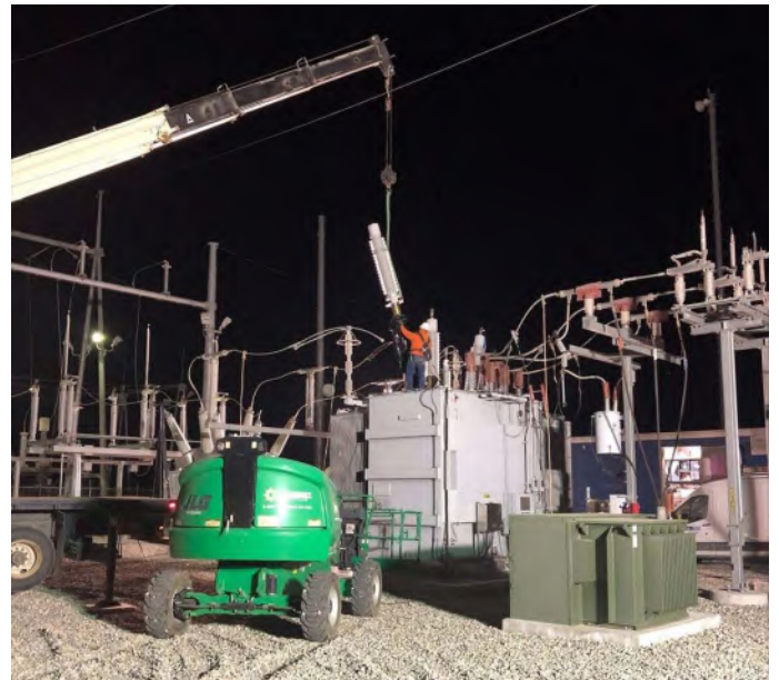
Figure 6. Night time H1 bushing replacement
