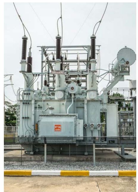
Figure 2. External type OLTC
