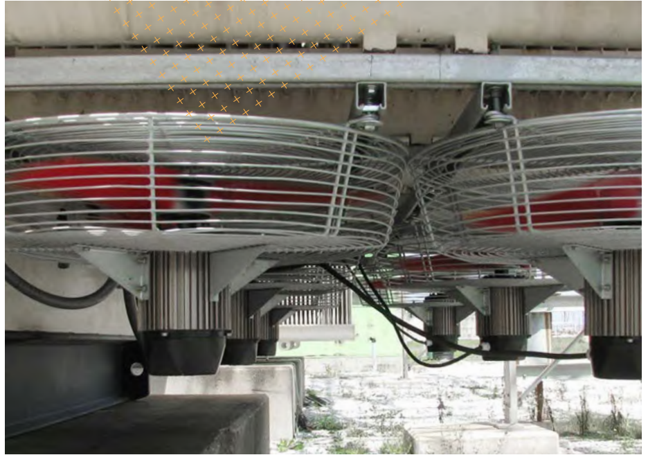
Figure 6. Unistrut bottom mount configuration
