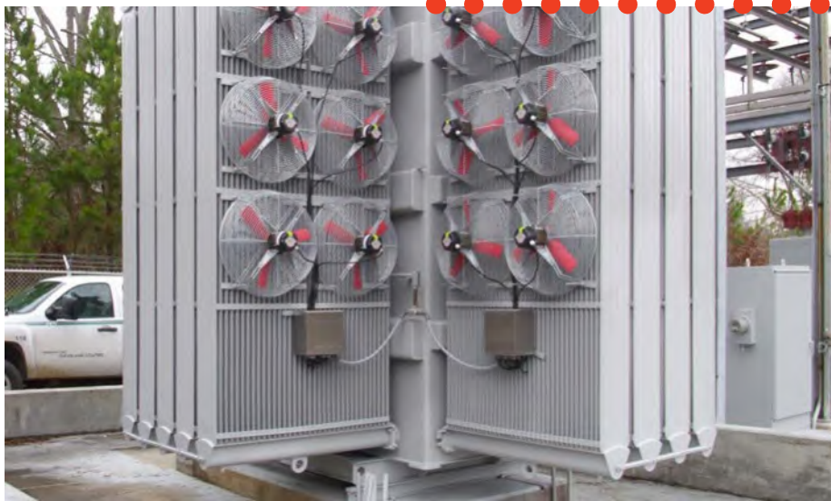
Figure 3a. Side mount airflow configuration
