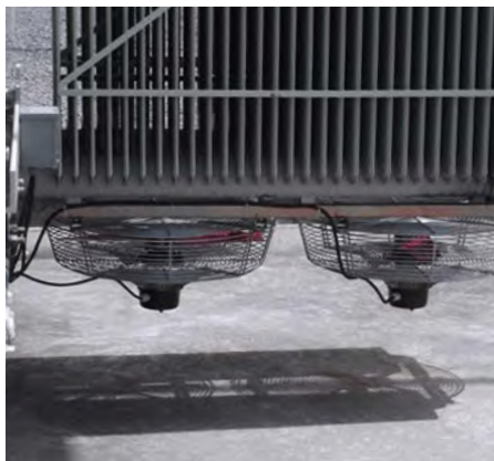
Figure 3c. Bottom mount airflow configuration
