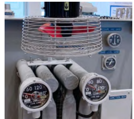
Figure 3e. Top mount airflow configuration
