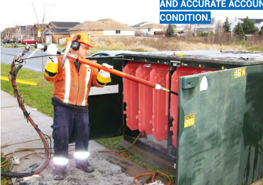
Figure 1. An electrical service technician applies simple dry ice cleaning on a residential transformer.
