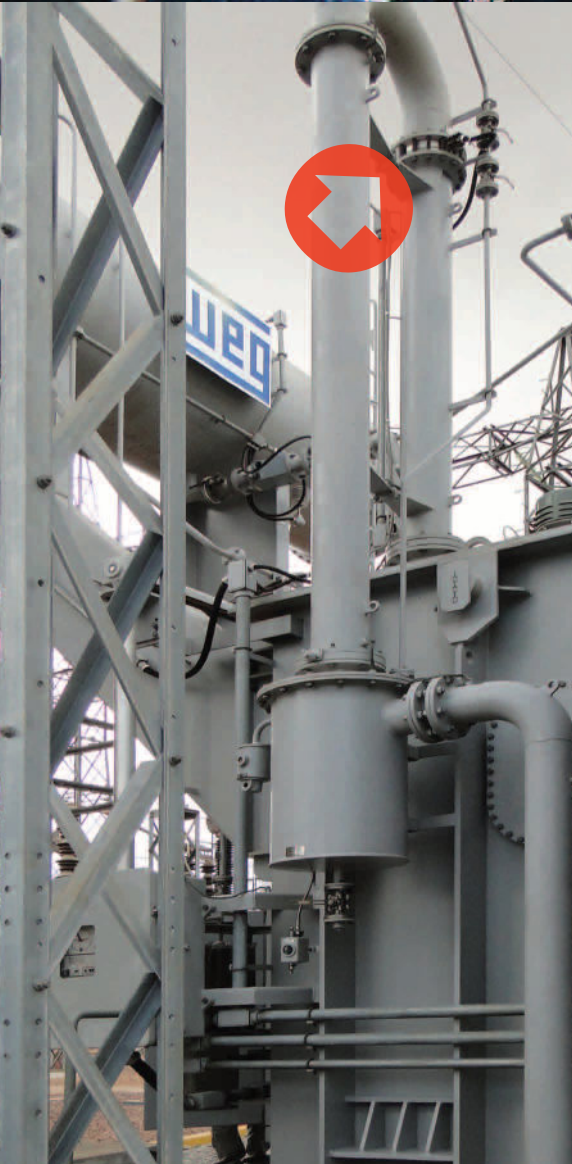
Figure 2. A ruptured disc in the confined discharge explosion tube in a 245/145-15 kV, 100 MVA autotransformer
