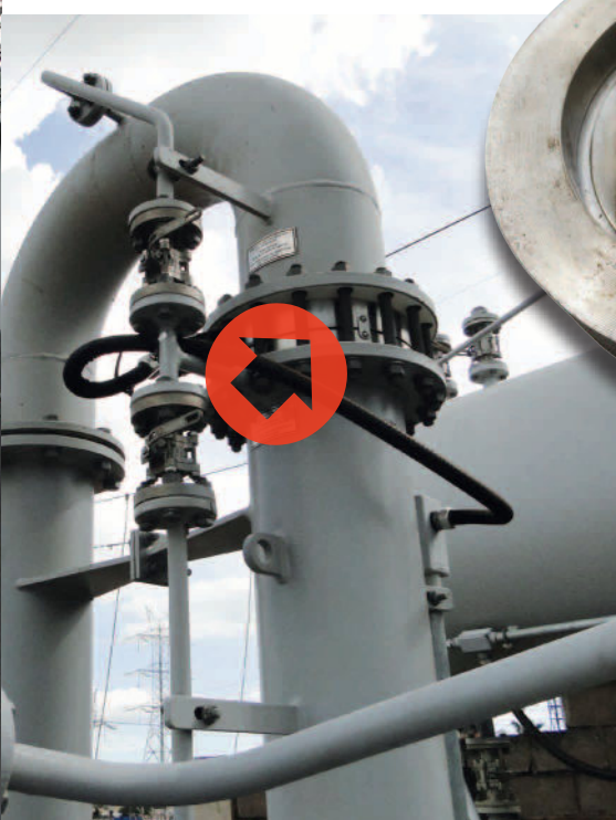
Figure 2. A ruptured disc in the confined discharge explosion tube in a 245/145-15 kV, 100 MVA autotransformer
