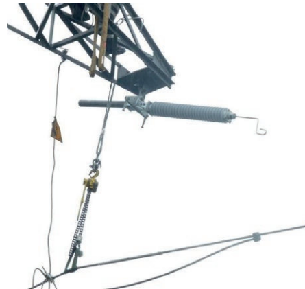
225kV EGLA – Installation in live conditions (1)
