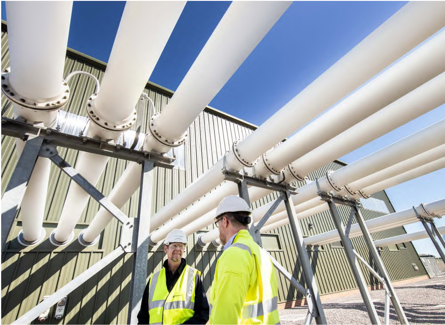
Hitachi Energy's EconIQ™ Retrofill replaces SF 6 in existing high-voltage equipment with an eco-efficient gas mixture.
