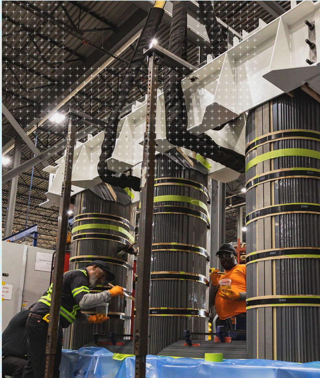
Applying Noise Reducing Epoxy on a Power Transformer Core
