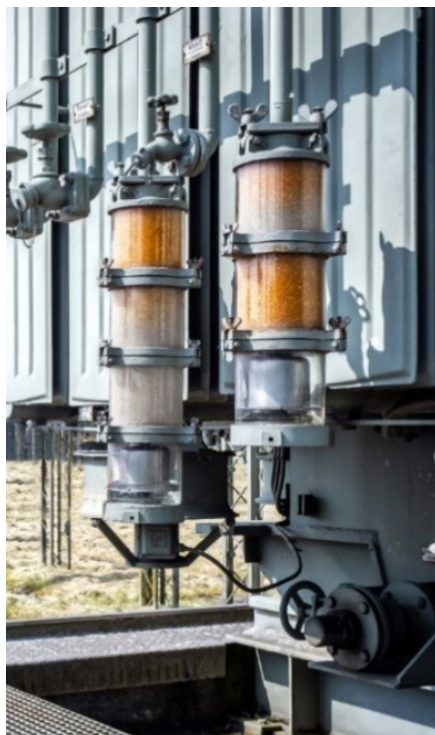
Conventional dehydrating breathers with color change from orange to colorless
