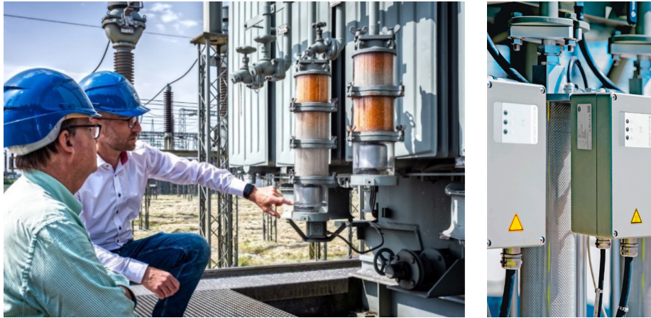
Comparison of a conventional (left) and a maintenance-free dehydrating breather (right).
