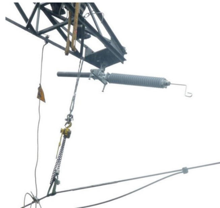
225kV EGLA – Installation in live conditions (1)
