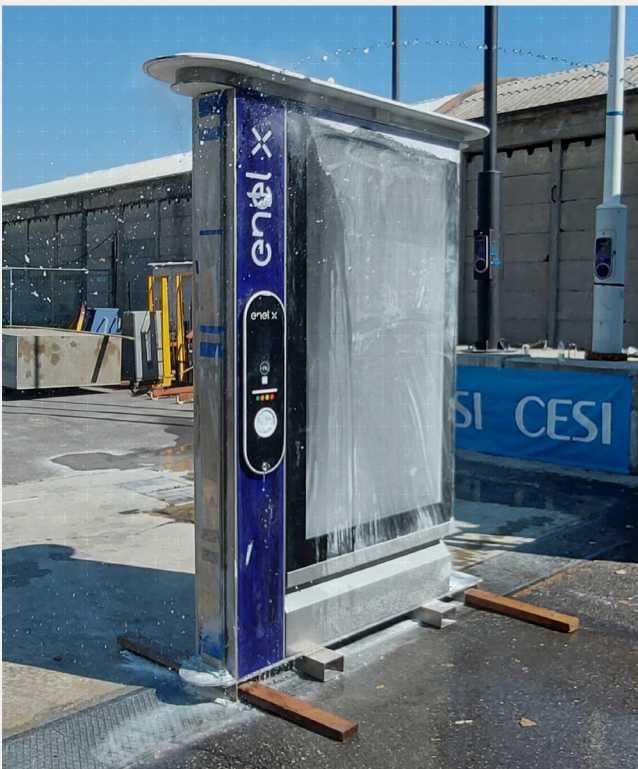
Water tightness test on charging column
